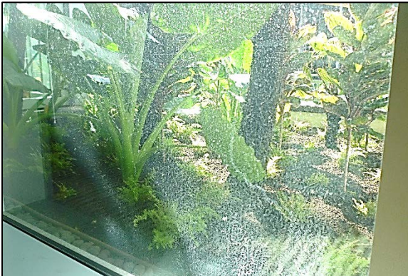
Scale on Glass Tower and Lofts
