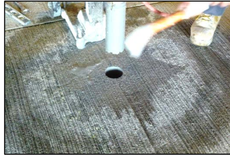
5 additional drains installed
