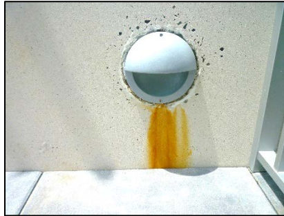
Rust and Red Dirt Removal Before
