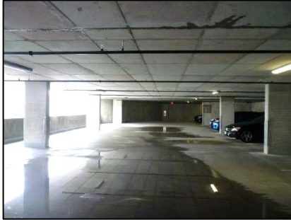
Ponding on Makai side of 6, 5 & 4 th floors
