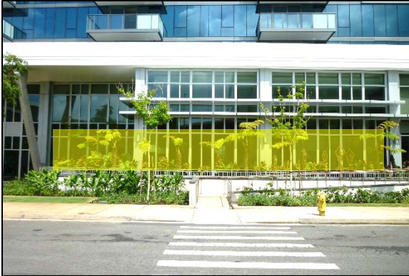
Keawe Street Tower
