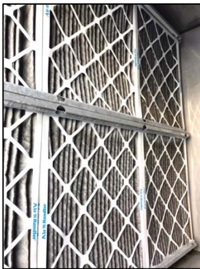
Filters needing replacement
