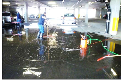
Ponding on Makai side of 6, 5 & 4 th floors
