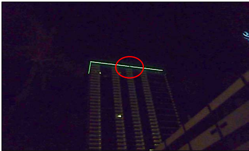
Section of Rooftop Parapet LED Ribbon Out. Work in Progress
