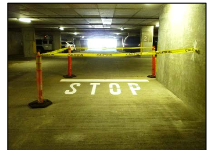
2/13/17 install of stop lines
