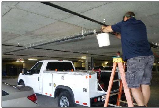
High Pressure Hose inserted into Storm Drain
