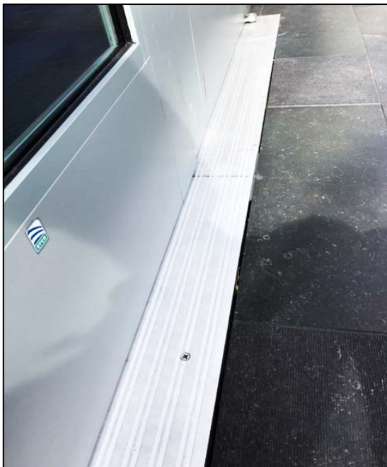
Gaps in Lobby Main Entrance Threshold subject to Water Intrusion (Motors are in threshold) Work in Progress
