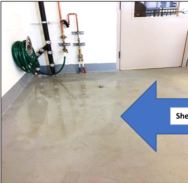
Dog Park: When Rinsing and Scrubbing, water flows away from the Drain. Work in Progress.
