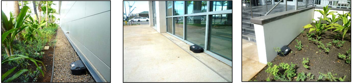
Bait Stations strategically placed around the project as well as the Rec Deck
