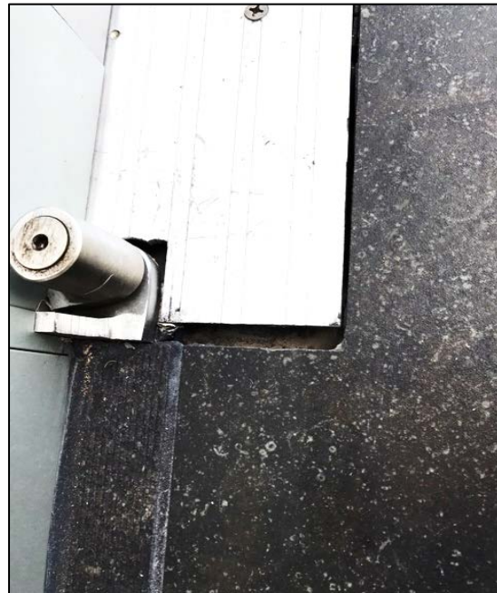
Gaps in Lobby Main Entrance Threshold subject to Water Intrusion (Motors are in threshold) Work in Progress
