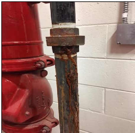
Leaking Fire Pump Plumbing Completed
