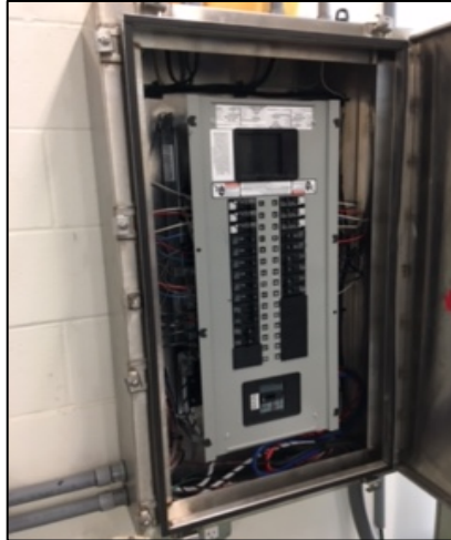
Exposed Energized Circuits Completed
