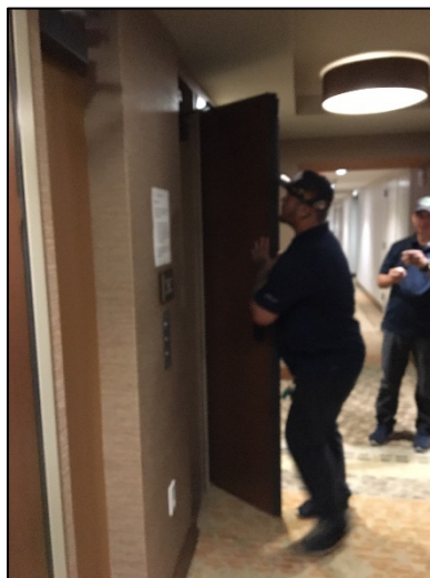
Defective door dragging on carpet
