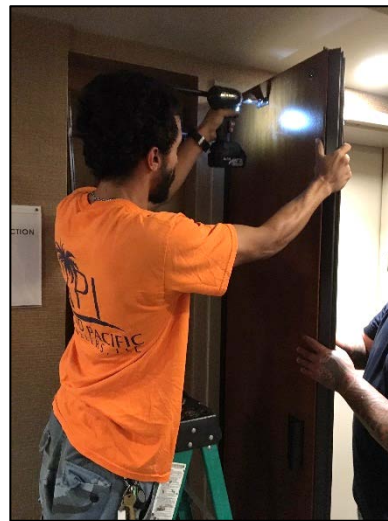
IPD performing repairs
