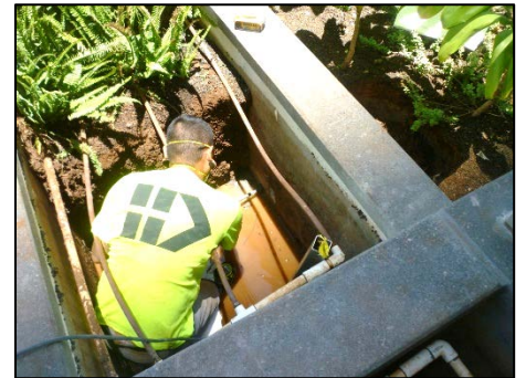
Larger Drains Drilled
