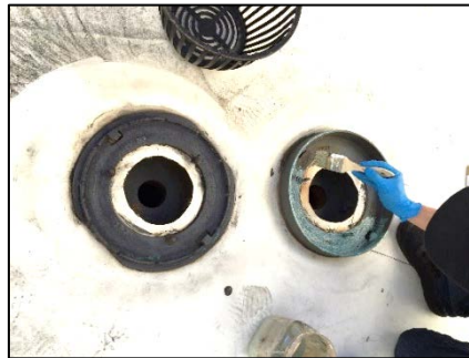
Corrosion Inhibitor application
