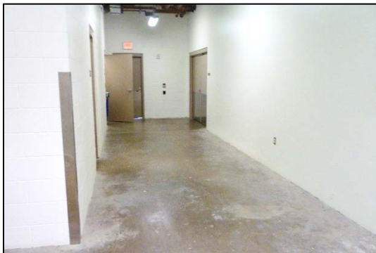
Before: Tower Trash Bin/Movers Corridor
