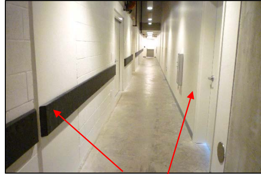
After: Crash Rails & Wall Protection
