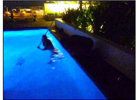
Pool Plaster Scrubbing
