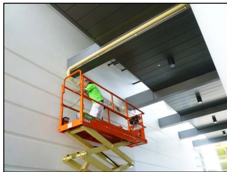
Storm Line being re-routed
