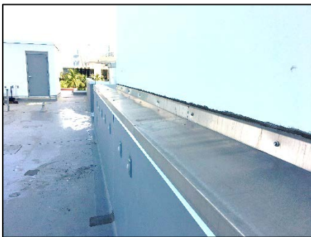
Lofts Flashing Before
