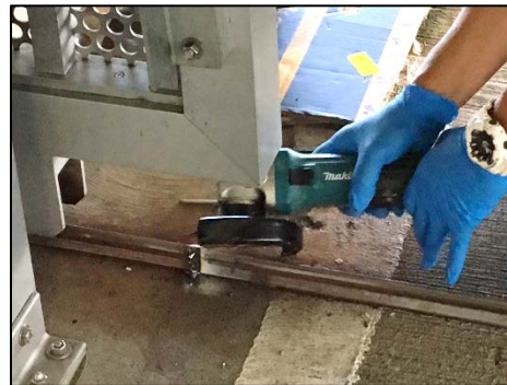
Grinding the weld flat for smooth gate operation
