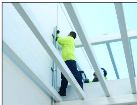
CPI Running Gas Line fr 6th to 7th fl
