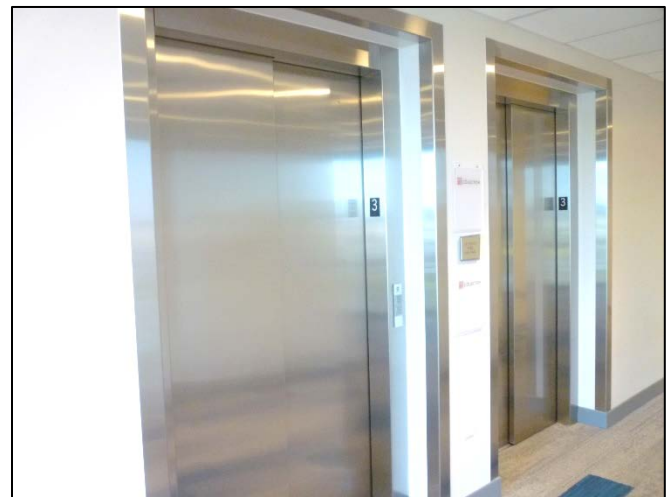
Stainless Steel Corner Guards added
