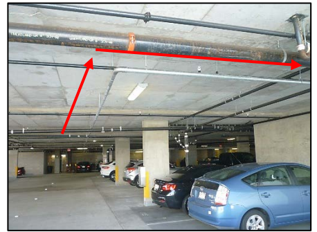
CPI Running New Gas Line to Pool Rm
