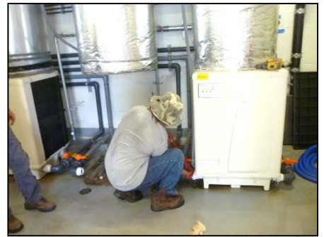
Removal of Existing Spa Heaters
