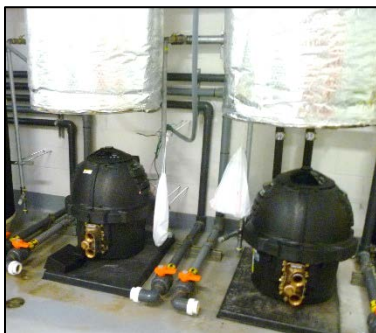
Placement of 2 of 3 Gas Heaters
