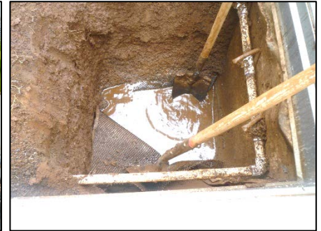
Installing Larger Drain
