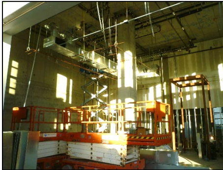
Duct work and fire sprinkler installation
