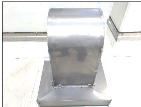
Tower Exhaust Hood After
