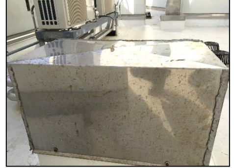
Tower Unit AC Penetration Box Before
