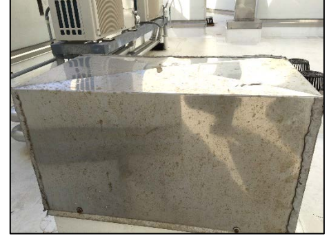
Tower Unit AC Penetration Box Before
