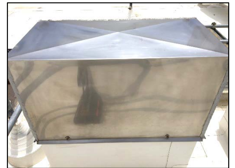
Tower Unit AC Penetration Box After
