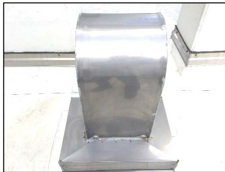
Tower Exhaust Hood After
