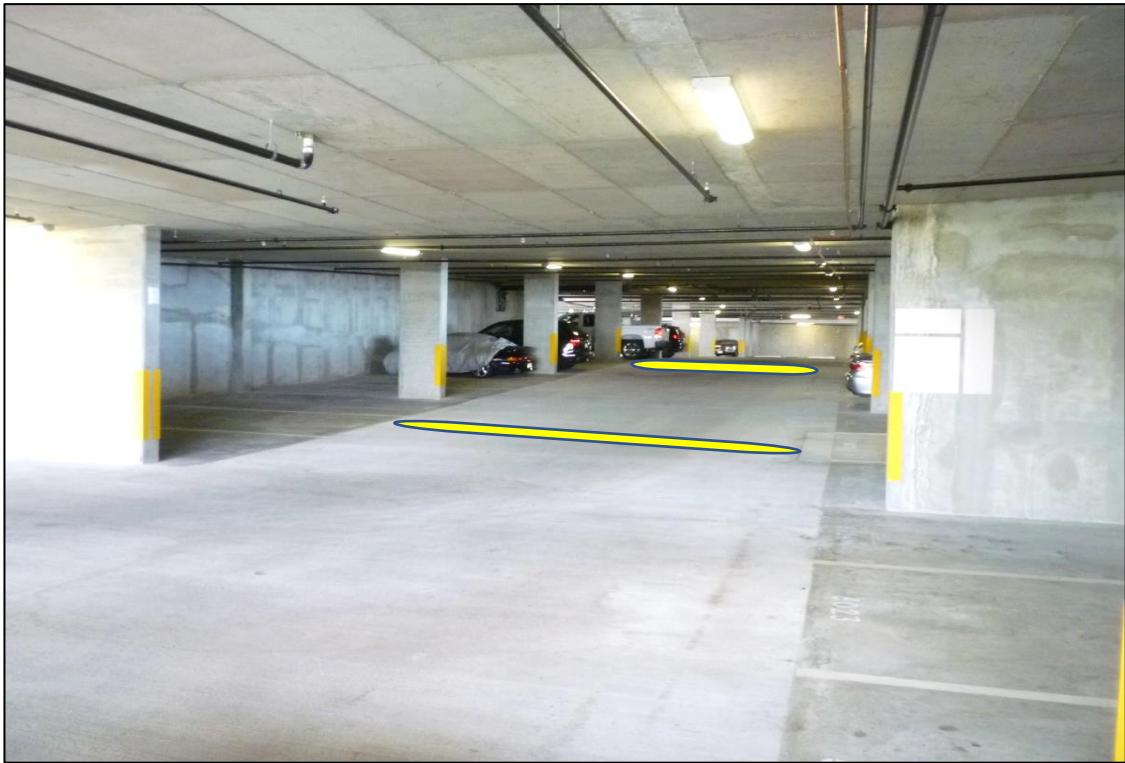
The Speed Bumps would be installed just before the turns. Installed enough distance prior to turns so both front tires arrive simultaneously Lengths will be long enough to prevent cars from going around them.
