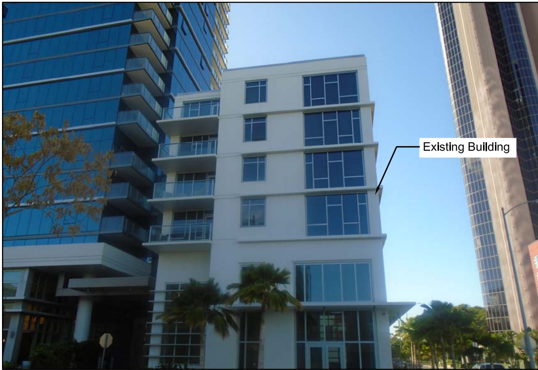
Looking Northwest Before
