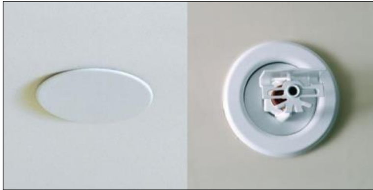
Concealed fire sprinkler in ceiling Standard fire sprinkler
